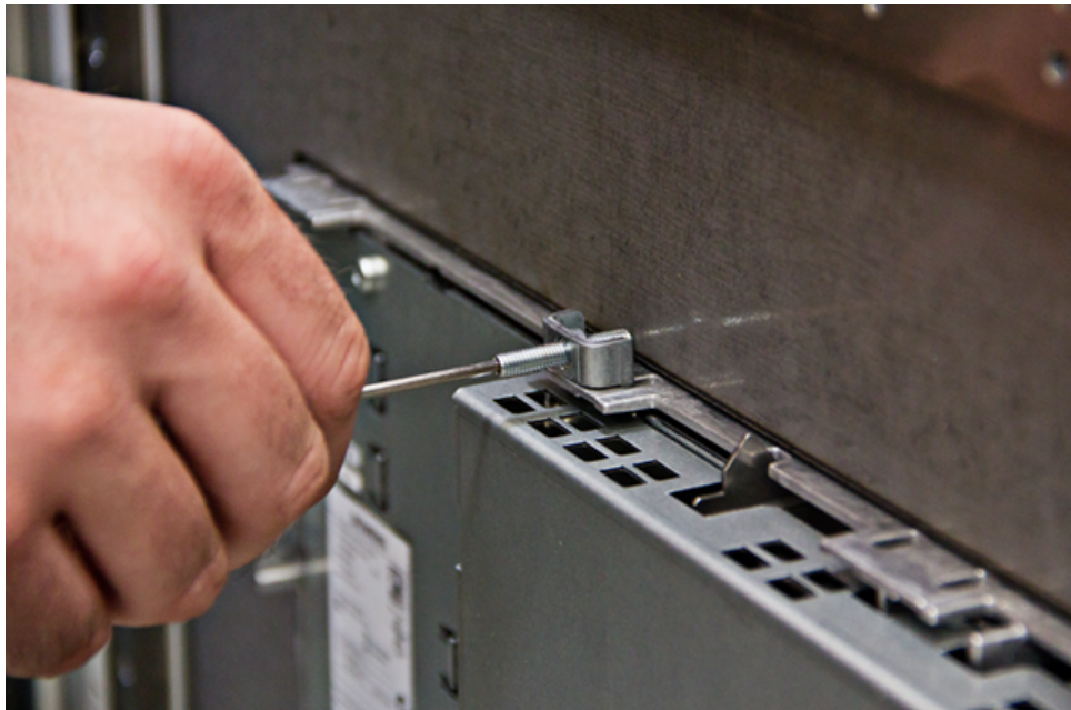
Image 11-6 Tightening the tension jacks
